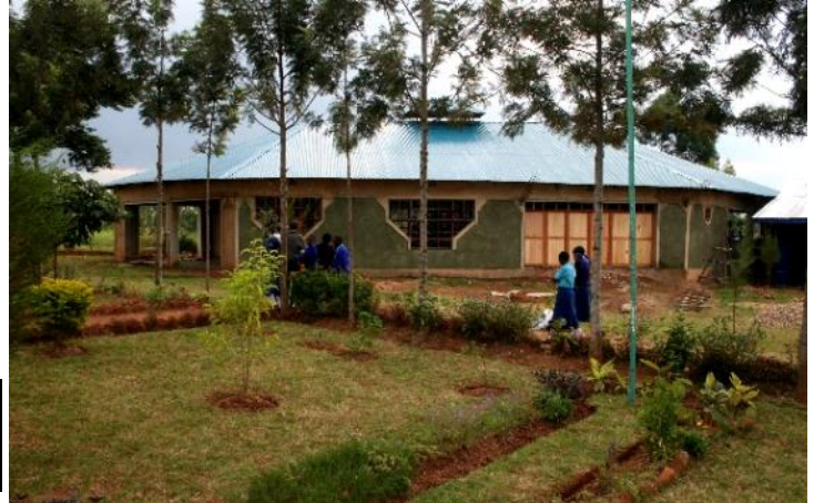
Mwituha Library is nearing completion!
