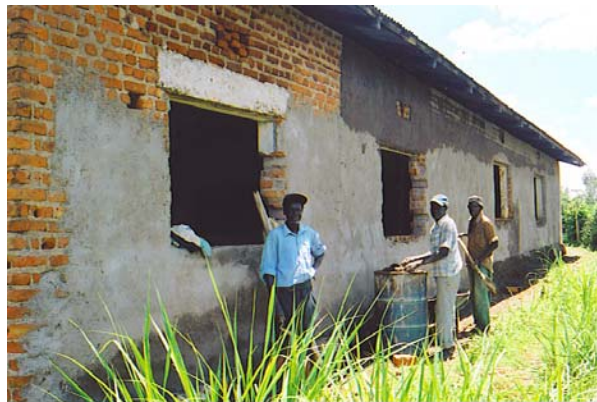
Refurbishing work for new classrooms.
