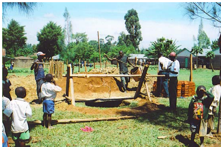
Well construction begins.
