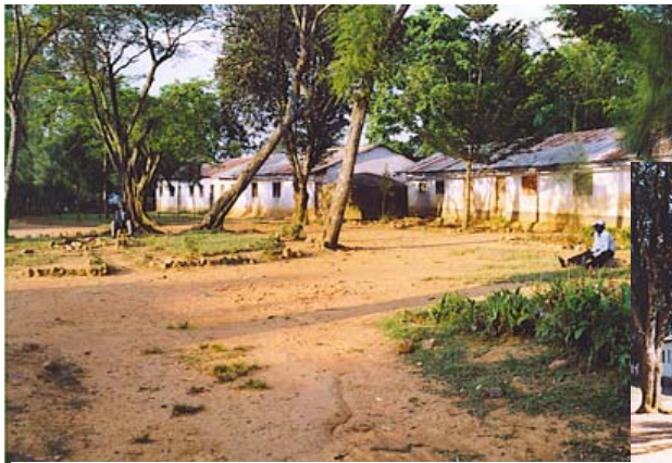
Essaba Primary School before the renovations.
